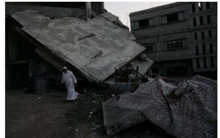
ALL PHOTOGRAPHS, PAUL FUSCO | MAGNUM PHOTOS A DANDY VAGABONDS™ 2010 PROJECT
